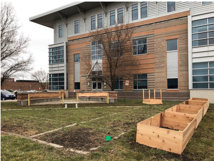
Installation of built accessible raised beds.
